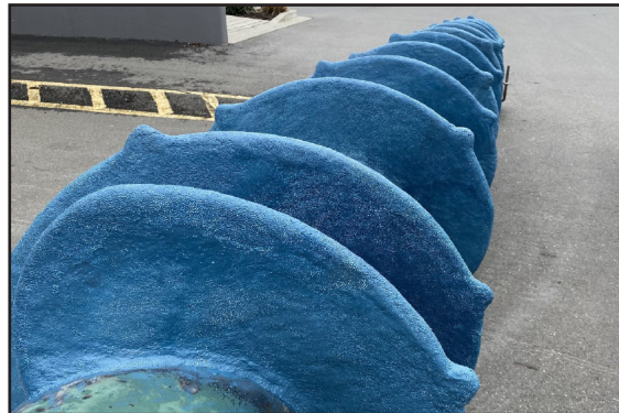
The screw surface with ARC MX1 industrial coating applied.
